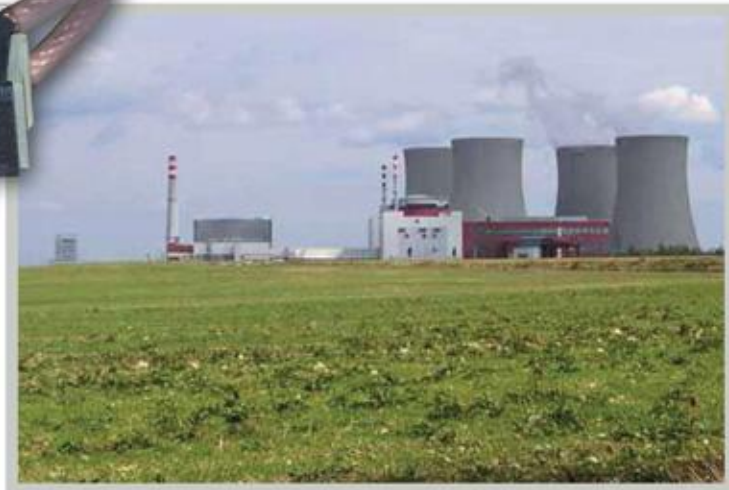
Temelin - nuclear power plant in the Czech Rep.
