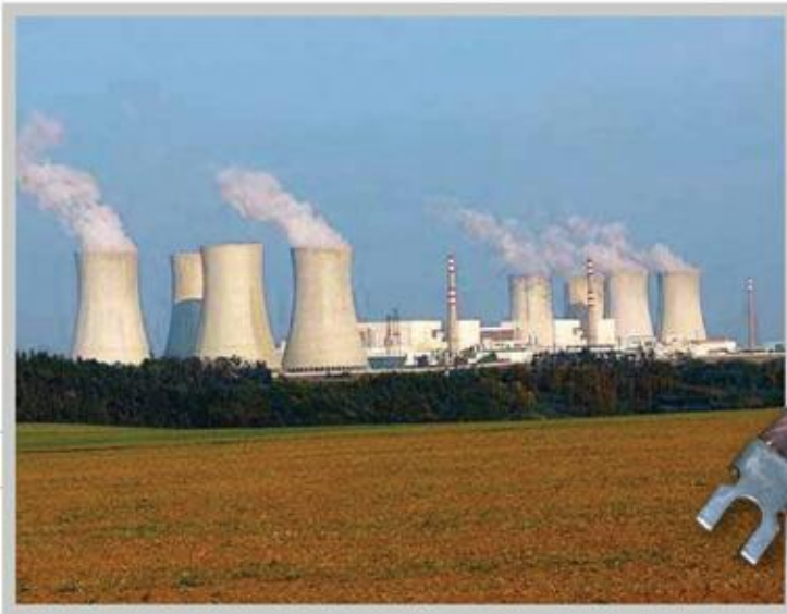
Dukovany - nuclear power plant in the Czech Rep.
